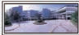
The City University of Hong Kong Division of Building Science and Technology BACnet Integration Points: 1,000+
